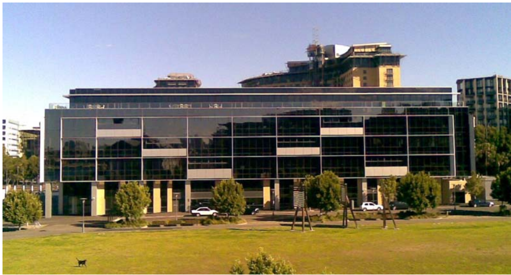
Figure 16: Workplace6 just finished in April 2009
